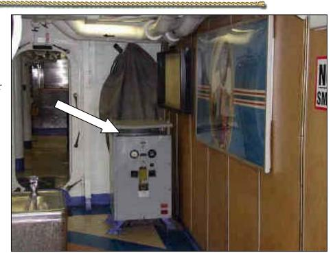
(ET) stationed at this position provides the 28Volt DC "juice" to the power cables seen on the helicopter maintenance cabin bulhead...
